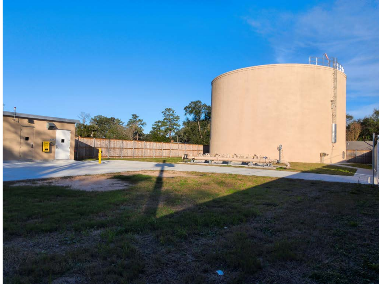
Water Plant #4 Tank Replacement
