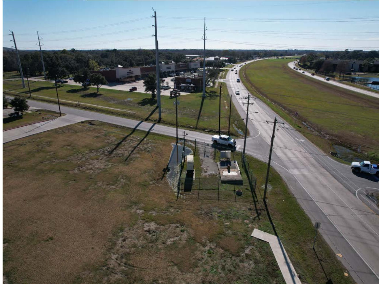
Lift Station #23 Expansion Project
