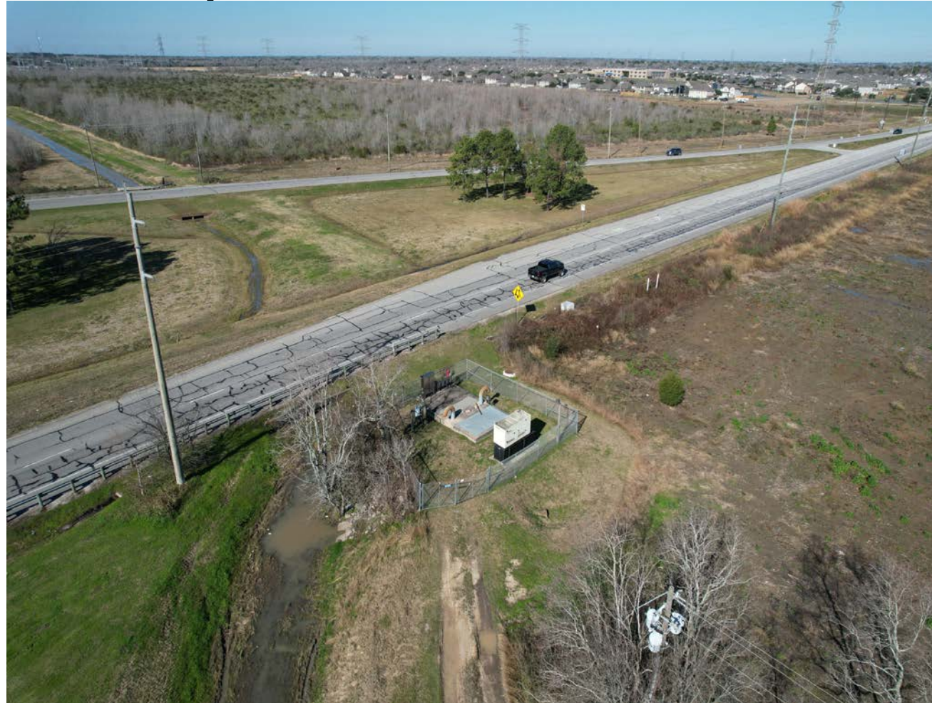
Lift Station #33 Rehabilitation Project
