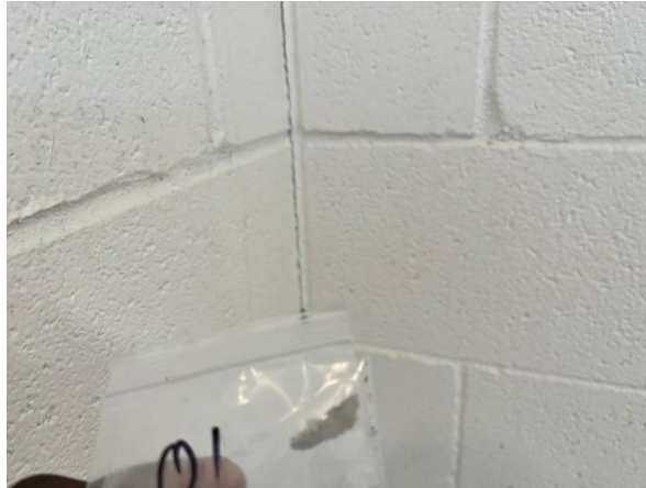
1. Sample #01 – cmu block mortar
