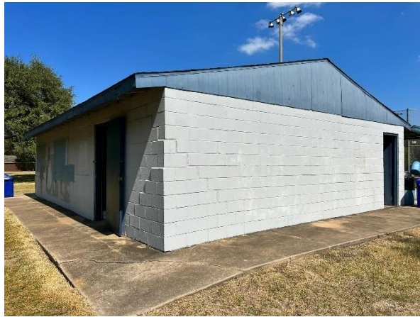
5. Exterior view at south side
