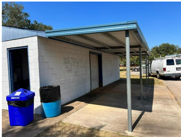
6. Exterior view at east side
