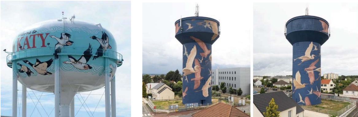
Figure 13: Example elevated water storage tanks with community identifying graphics
