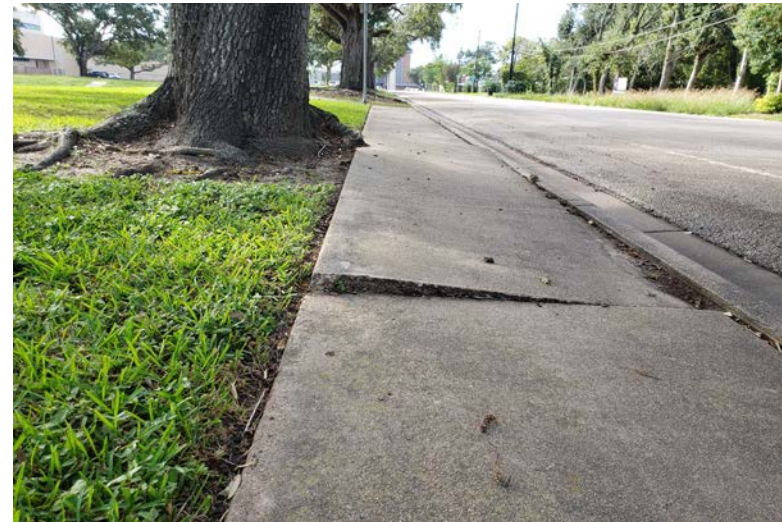
📍 Grade separation on existing sidewalk
