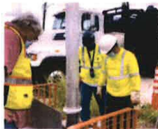
Lift Station Cleaning
